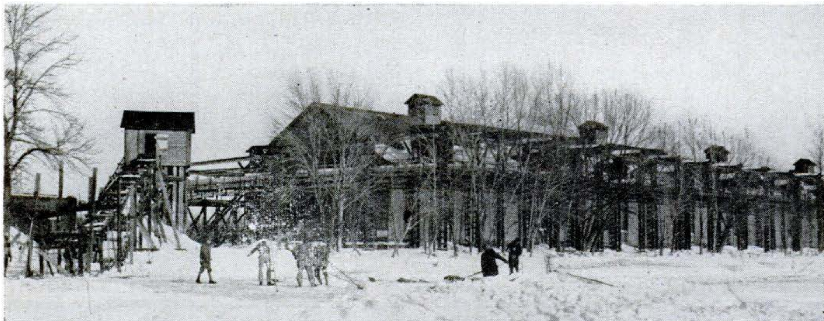
1. Icehouse has capacity of 7,000 tons. At far left is inclined conveyer that lifts the cakes to moving gallery. This runs outside the
